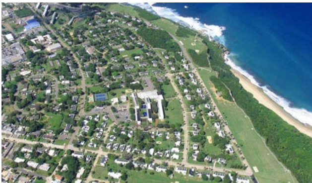
FIGURE 2: Aerial View of Installed PVs
